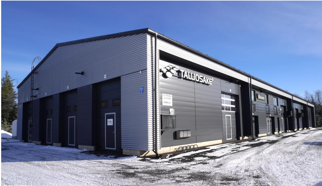
Photo 1. The building of Herukan Talliosake Oy at Varsikuja 7. The facade faces Varsikuja.
